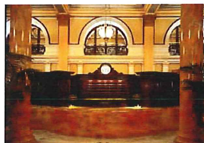
After rehabilitation, this severely deteriorated space was returned to its original elegance. Plaster was repaired and repainted; scagliola columns were restored to match marble; and missing decorative metalwork was re-installed in front of the windows. Photo: Carol M. Highsmith.
