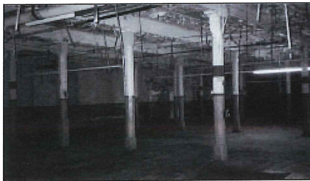
Exposed structure of the mill building prior to rehabilitation.
