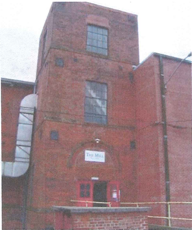
Main Mill South Side
