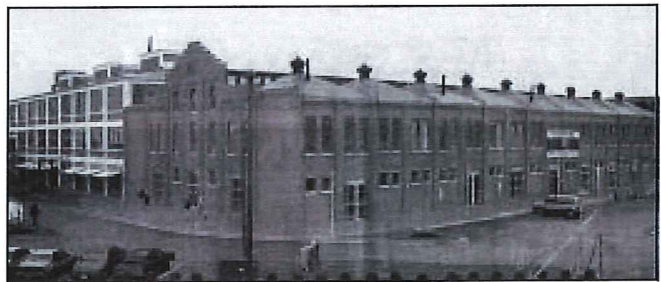
Tin can factory following rehabilitation.
