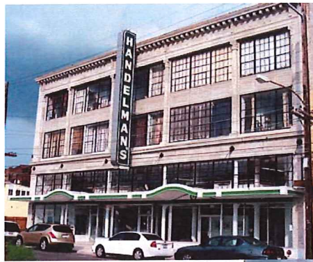
Left: This three-story building (shown after rehabilitation) was constructed in 1923 for use as a department store.
